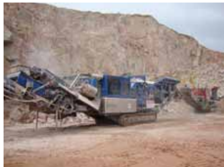
Bandwaage in mobiler Brechanlage
